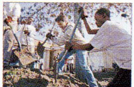
John Edwards shovels with student volunteers as he works at a house in an area affected by Hurricane Katrina in New Orleans.
